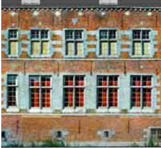
Figure 8 : Façade extérieure (Est)
